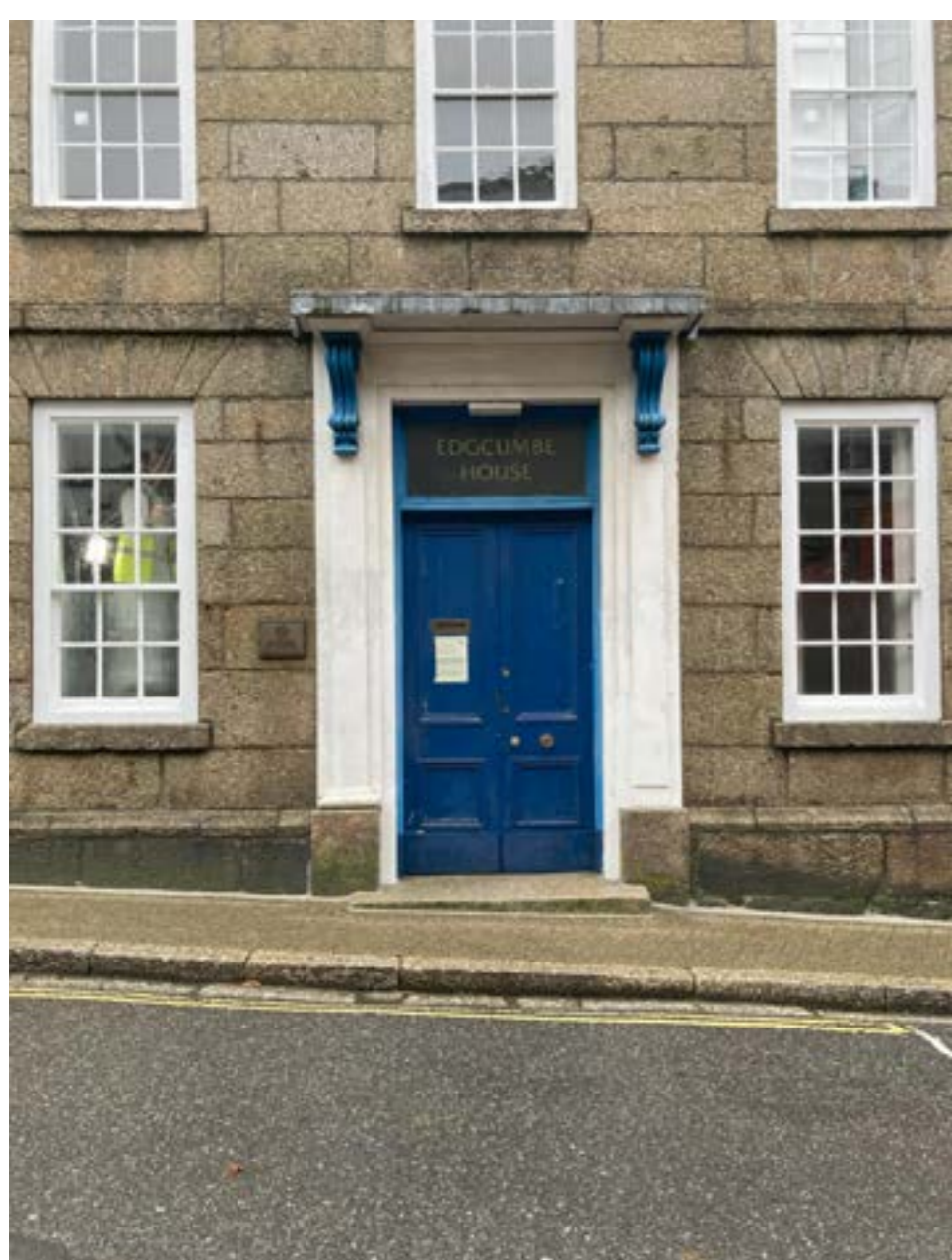
Fore Street Elevation of Edgcumbe House
