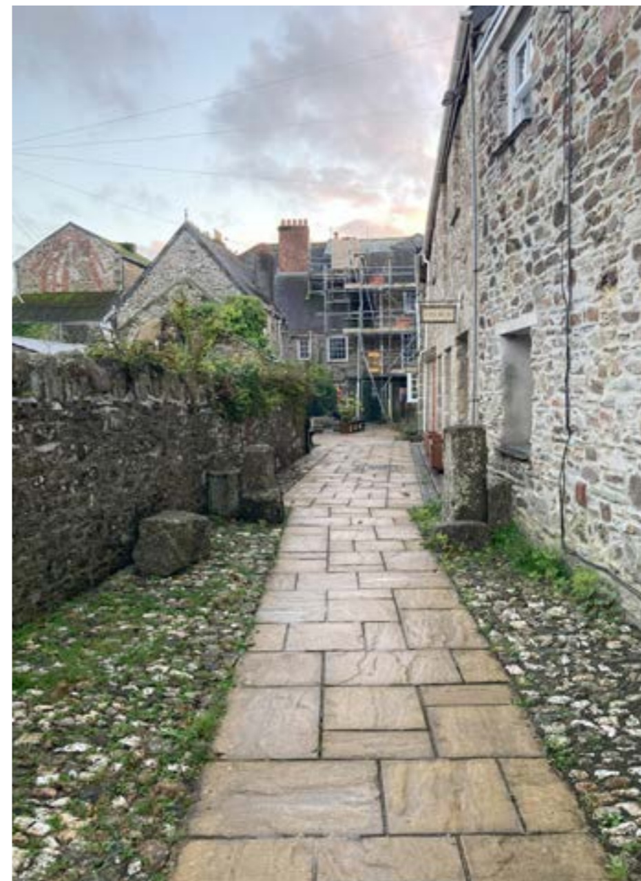
Existing Access to Taprell House and Rear of Edgcumbe House
