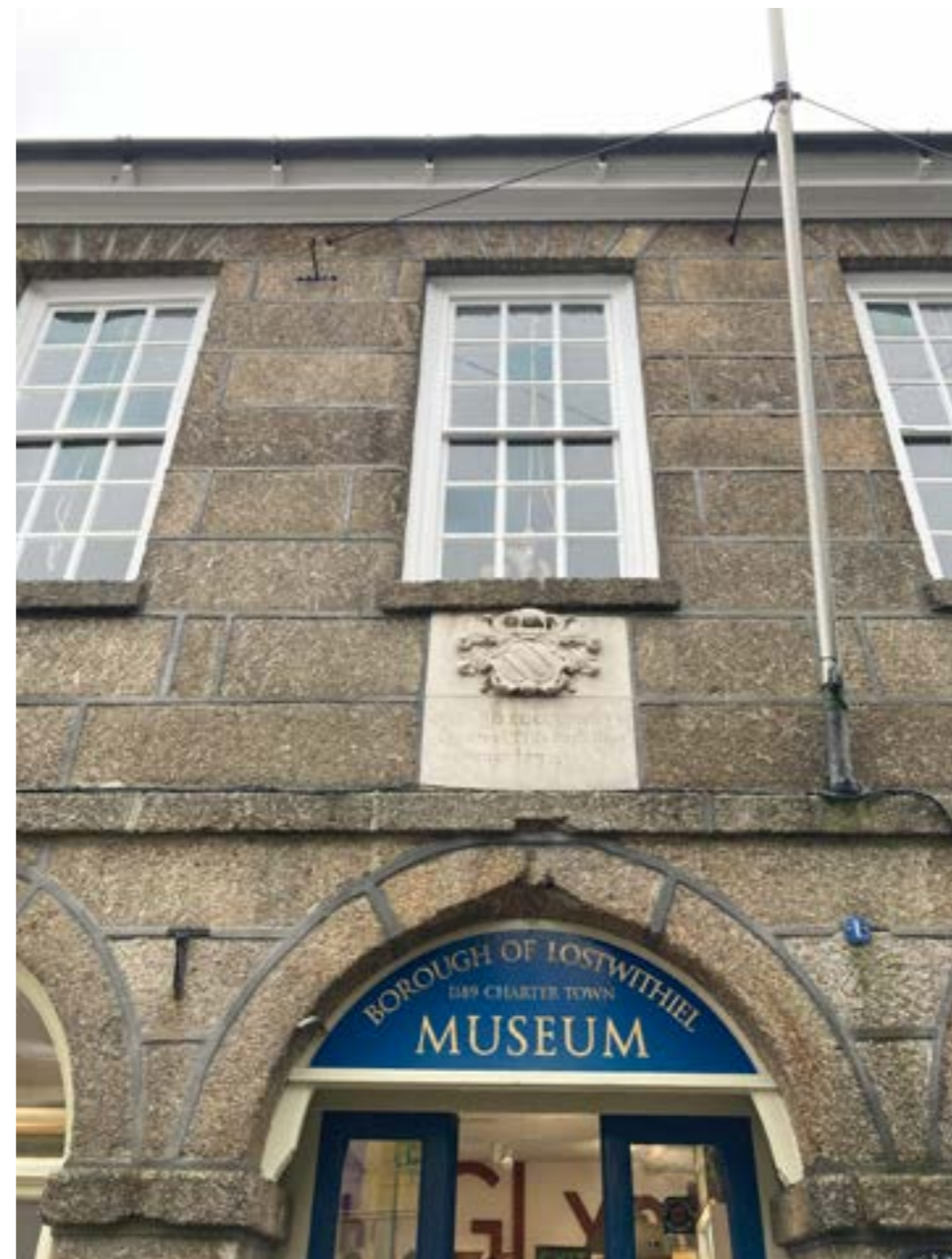
Fore Street Elevation of Museum / Guildhall
